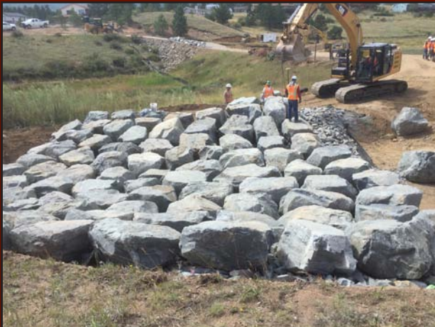
Carriage Hills Dam Repair Project - West Dam Spillway
