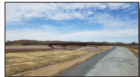
The completed Sandstone pedestrian bridge (right).
