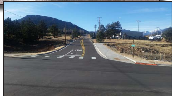
Above: Brodie Avenue at Fish Creek during the 2013 flood Below: Brodie Avenue at Fish Creek after 2017 repairs
