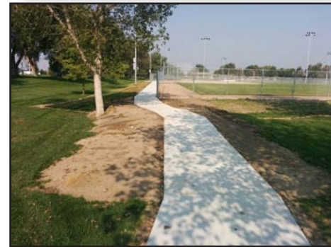
2018: Trails have been repaired and an ADA sidewalk built in the park.
