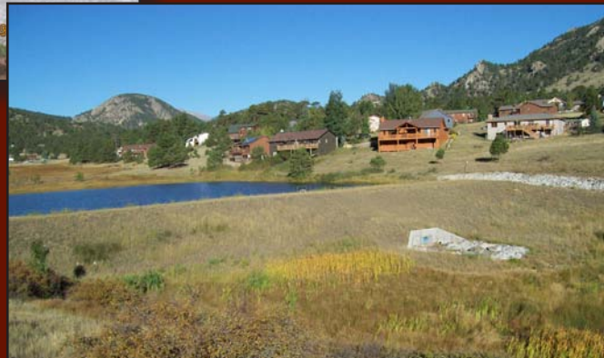
Above, left: Carriage Hills West Dam during the flood
